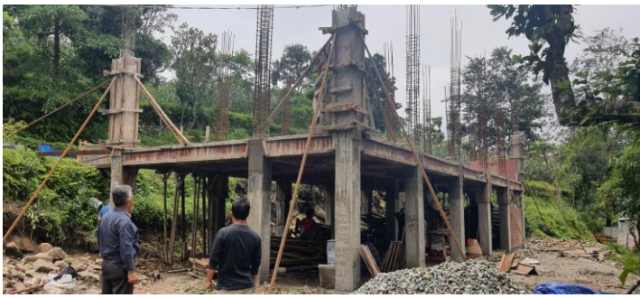
The completed slab and column casting of 1 st floor at Sotang hostel construction project site
