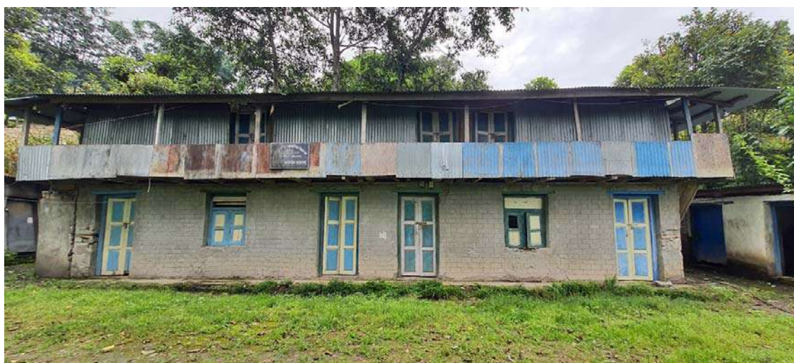
Existing hostel building condition of Sotang School
