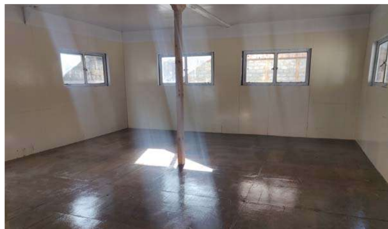
➤ The internal part of the completed first phase of the renovation.
