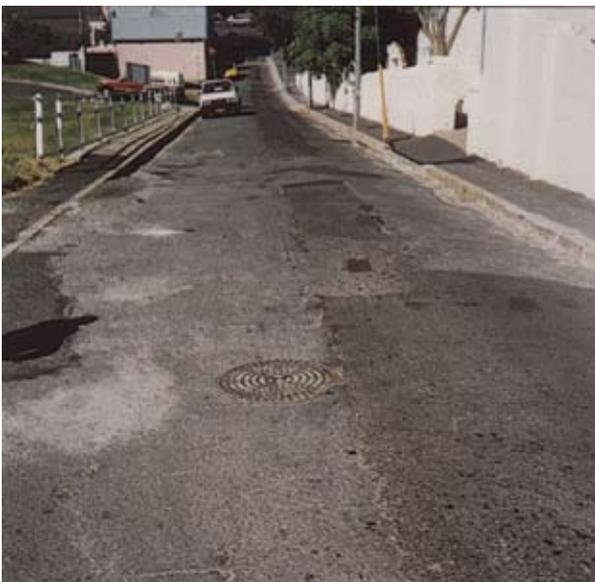
**Photograph 8** – Upper Rhine Road - section still to be rehabilitated
