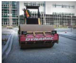
Base construction uses locally available materials. Pavers are delivered ready to place, joints filled, compacted and ready for traffic.
