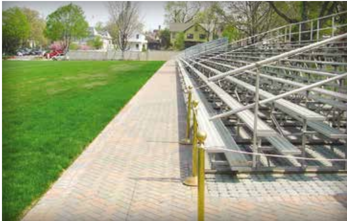
PICP under bleachers at the U.S. Naval Academy in Annapolis, MD provides structural support and on-site infiltration.
