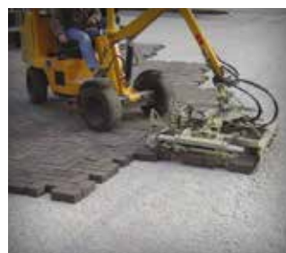
Mechanical installation equipment accelerates construction; typical 5,000 sf (500 m 2 )/machine/day. After placement, joints and/or openings filled with small aggregate and pavers are compacted.
