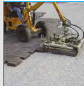
Mechanical installation speeds construction. Aggregate base and subbase are spread and compacted; pavers are delivered ready to install. After placement, joints and/or openings are filled with small aggregate and pavers compacted at this Walmart in Rehobeth Beach, DE.
